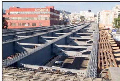
*Central Viaduct, San Francisco, CA. A 10-span, 1,422-foot-long, continuous girder structure with integral concrete bent caps. It replaces a segment of an existing viaduct, and is being constructed while remaining open to the street traffic underneath.*
