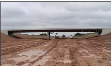
Missouri's first completed High-Performance Steel (HPS 70W) bridge, a two-span, five-girder structure located at Route 224 over future Route 13 in Lexington.
