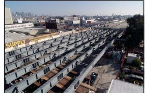
*Central Viaduct, San Francisco, CA. Girders are hybrid, flange — A 709 HPS Grade 70W and web — A 709 Grade 502. Bridge is currently under construction and is expected to be completed by May 2005.*
