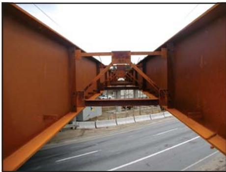
*Typical intermediate cross frames consisted of K-frames with a bottom chord. High-performance steel and weathering steel was used throughout the structure.*
