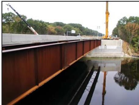
*The Route 3 Northbound Bridge over the Concord River in Billerica, Massachusetts is a 220-foot long single span bridge with 8-foot deep hybrid plate girders. Grade 70 High-Performance Steel was used on both the top and bottom flanges in the center 118-foot sections.*
