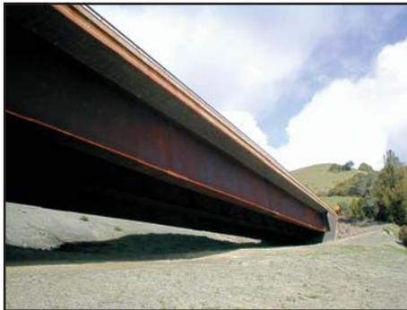
The Whites Hill Sidehill Viaduct, Marin County, CA. A 380-foot-long, 43-foot-wide, 14-foot seven-inch deep, three-girder, single span bridge.
