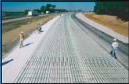
One such study, an interstate highway corridor in South Dakota constructed between 1962 and 1974, used doweled jointed reinforced concrete pavement (JRCP), asphaltic concrete pavement (ACP), continuously reinforced concrete pavement (CRCP), and full-depth asphaltic concrete pavement (FDACP).
