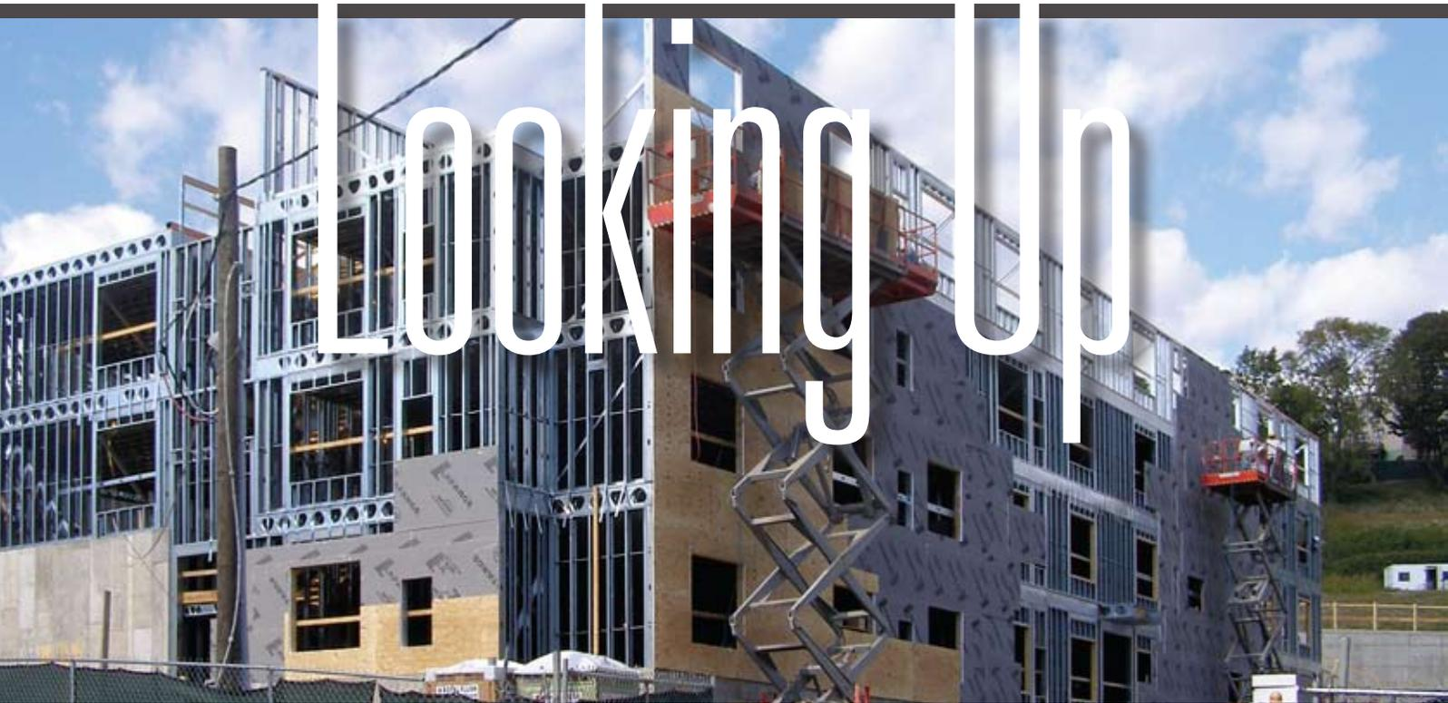
Each piece of cold-formed steel was ordered cut to length, including the 6-inch wall studs, by MarinoWARE, South Plainfield, N.J.
