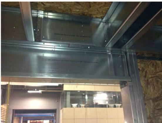
(a) typical header, ledger, and joist
