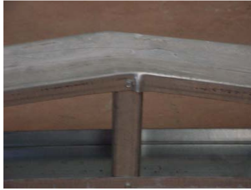
Figure 4.13 – Failure of Specimen 3D24-16
