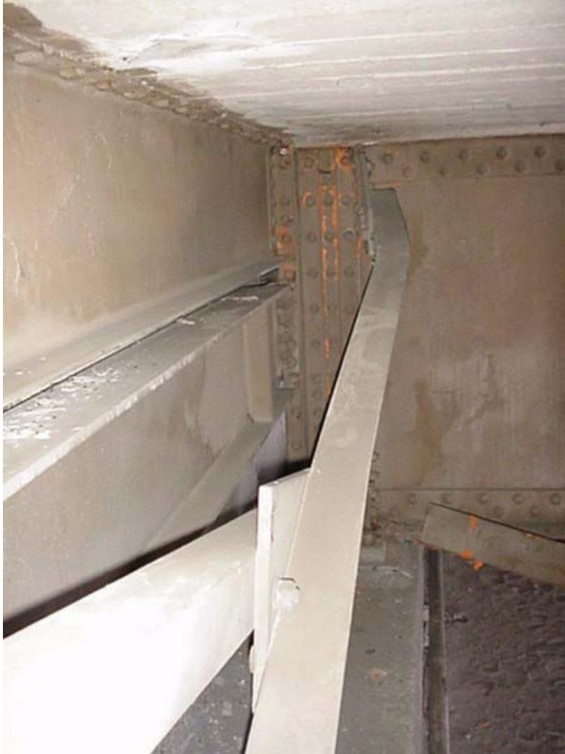
Figure 1-166. Buckled end cross frame member in Capitol Arch Bridge during the 2001 Nisqually Earthquake in Washington.
