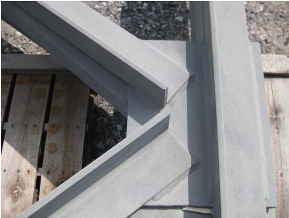
Figure 1-16. Details of cross frames with inverted V-pattern diagonals
