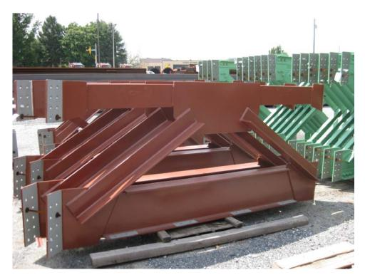
Figure 1-11. Abutment cross frames with V-pattern diagonals
