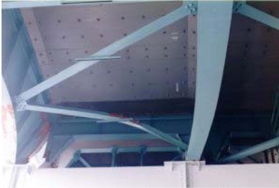
Figure 1-7. Damage to End Cross Frames and Girders during 1995 Kobe Earthquake.
