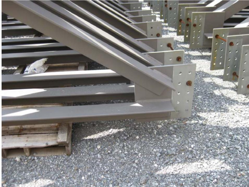
Figure 1-19. End details of cross frames with X-pattern
