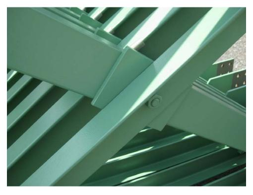
Figure 1-23. Middle details of bolted cross frames with X pattern
