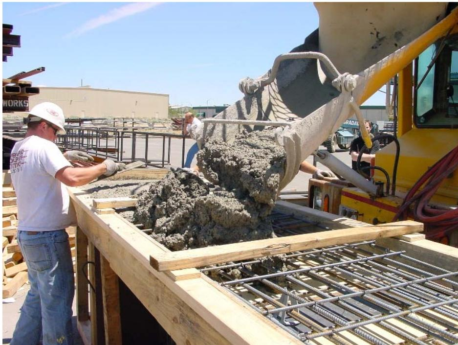
Figure 1-71. Pouring concrete for Specimen F1C
