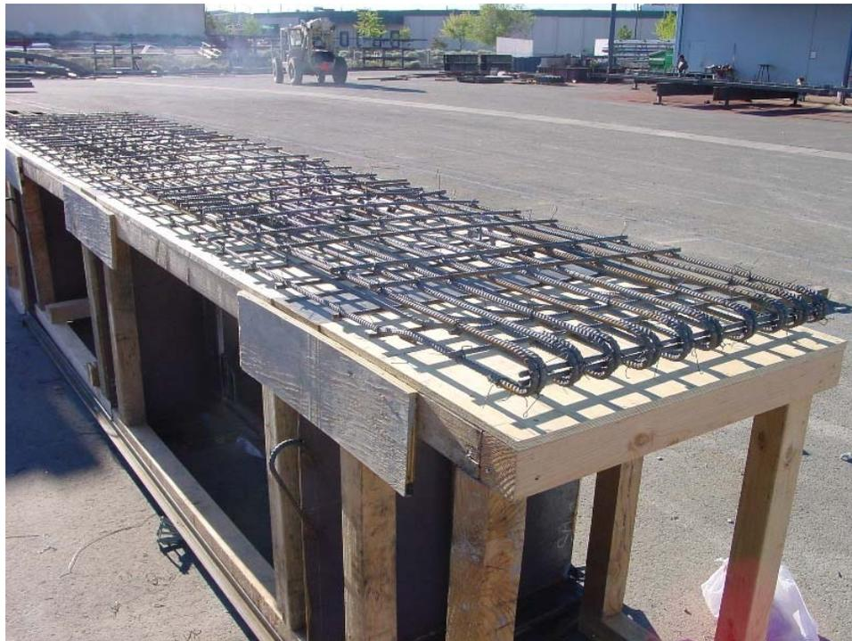
Figure 1-67. Rebar arrangement for Specimen F1C
