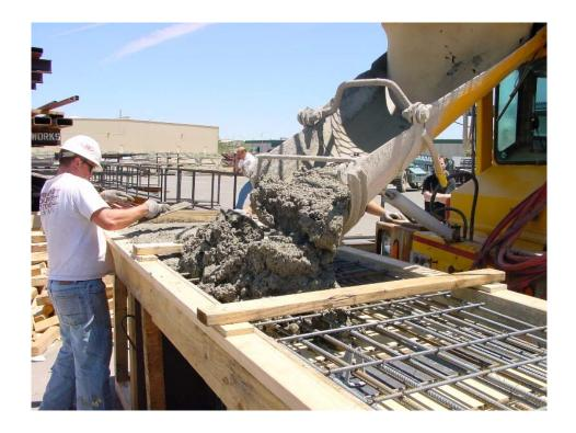
Figure 1-71. Pouring concrete for Specimen F1C
