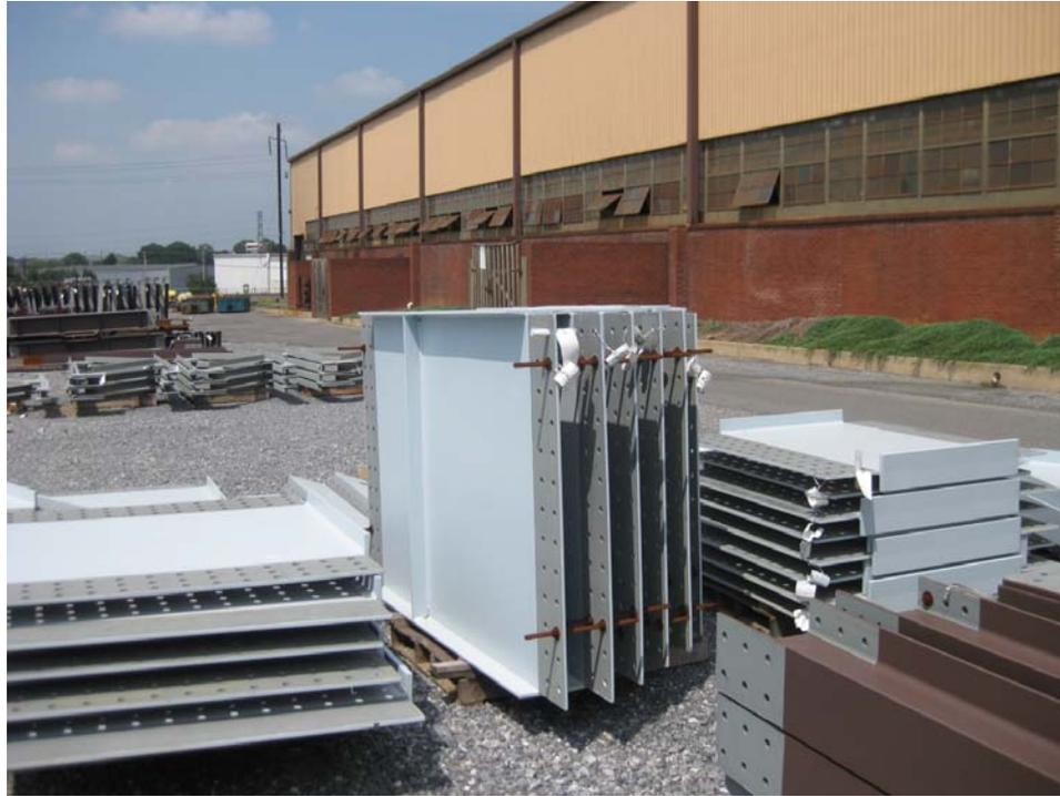
Figure 1-13. Built up I-section diaphragm with transverse stiffener
