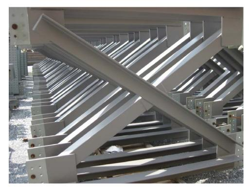
Figure 1-18. Details of cross frames with X-pattern diagonals
