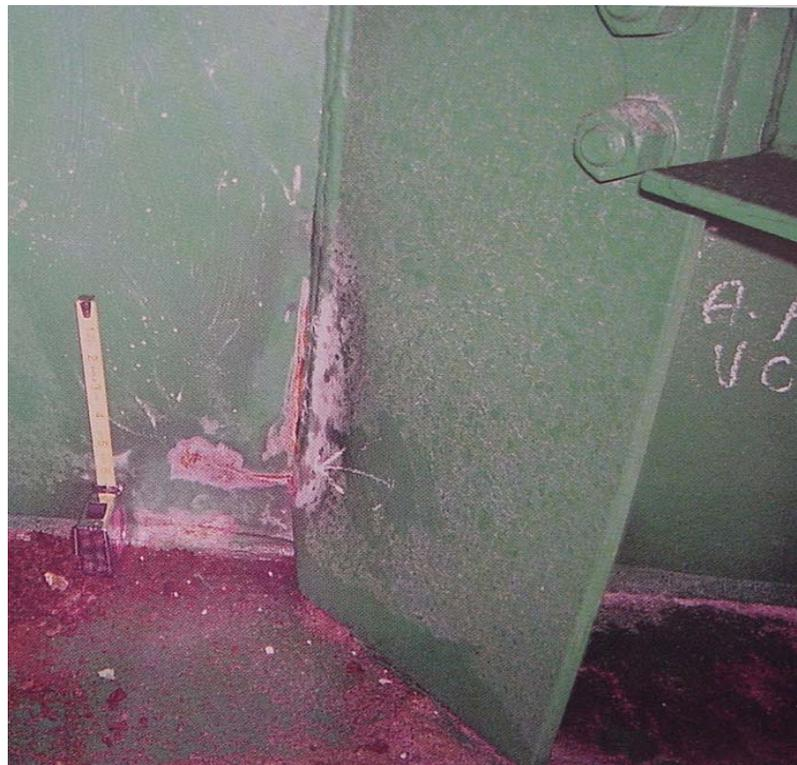
Figure 1-6. Damage to Web Stiffeners during the 1994 Northridge Earthquake.
