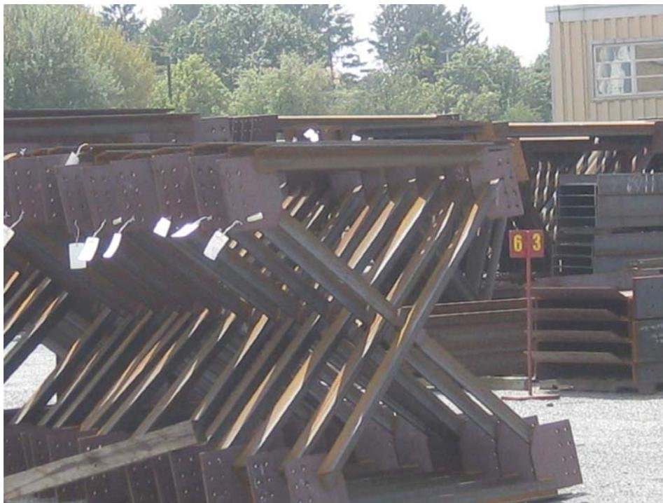
Figure 1-10. Bent cross frames with X-pattern diagonals
