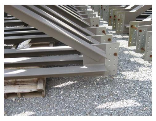
Figure 1-19. End details of cross frames with X-pattern
