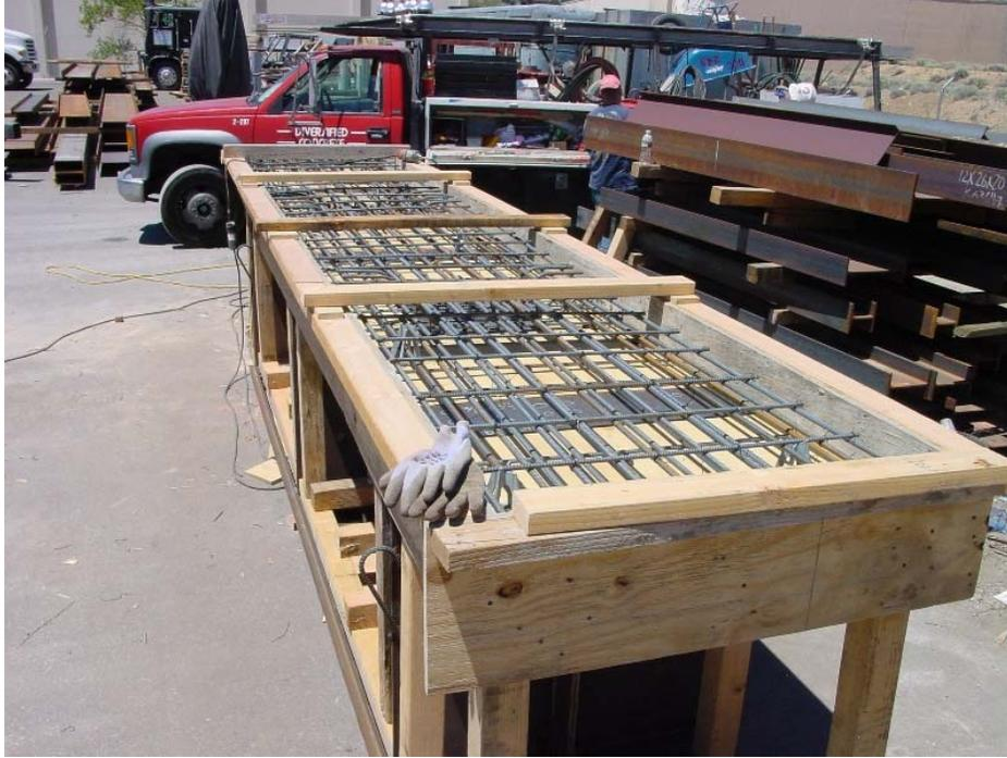
Figure 1-70. Specimen F1C: completed rebar and formwork
