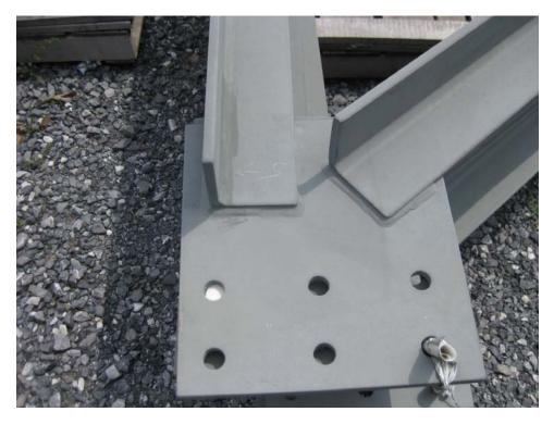
Figure 1-17. End details of cross frames with inverted V-pattern
