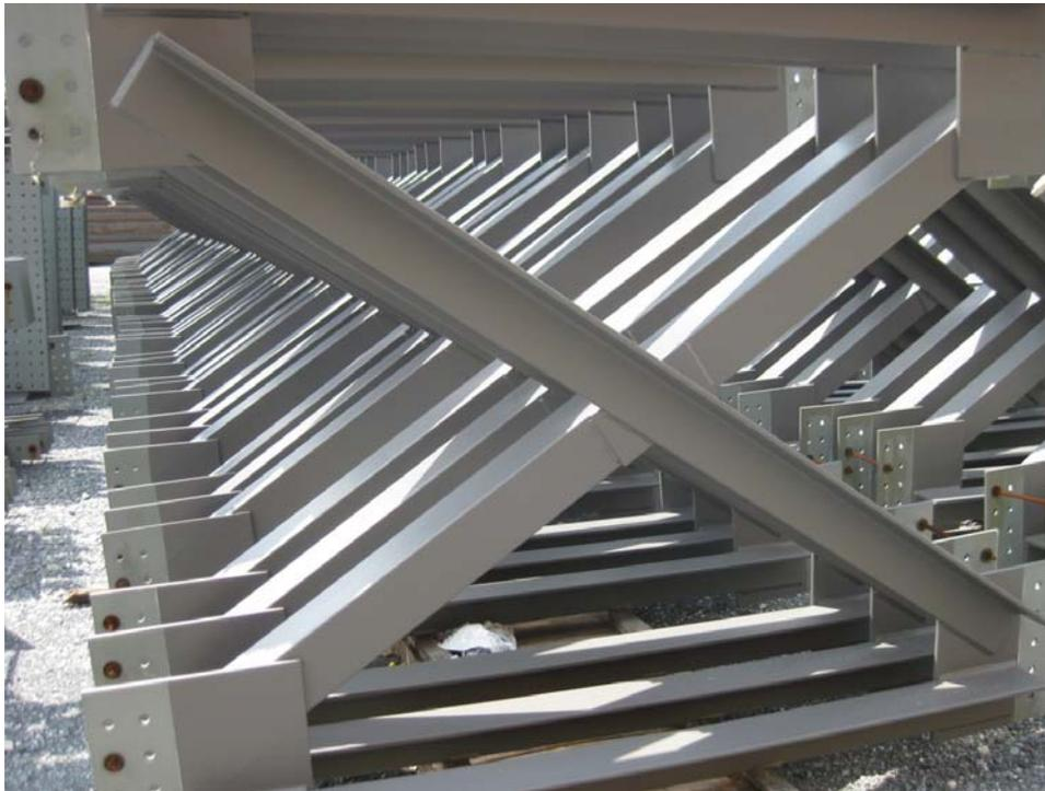
Figure 1-18. Details of cross frames with X-pattern diagonals
