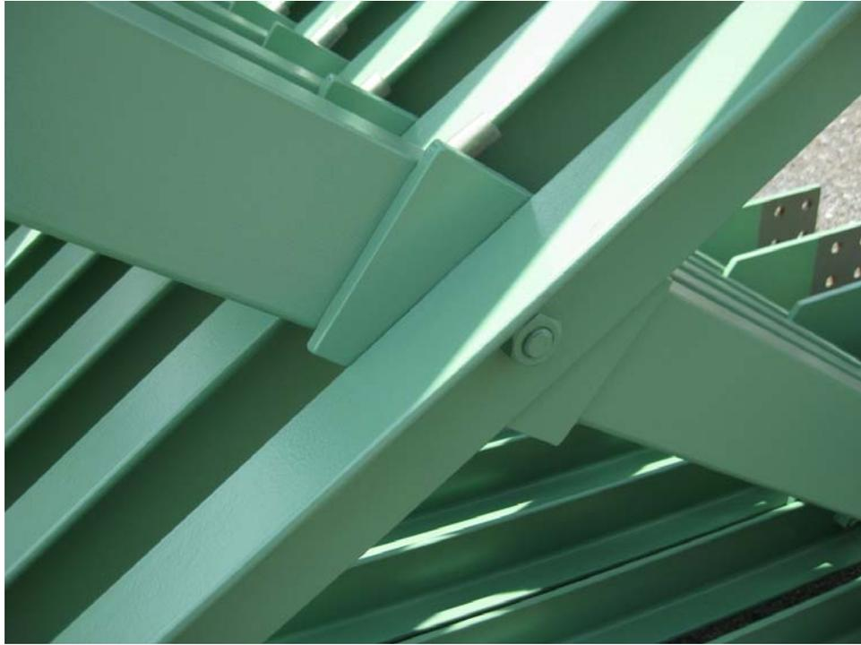
Figure 1-23. Middle details of bolted cross frames with X pattern
