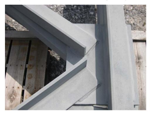
Figure 1-16. Details of cross frames with inverted V-pattern diagonals
