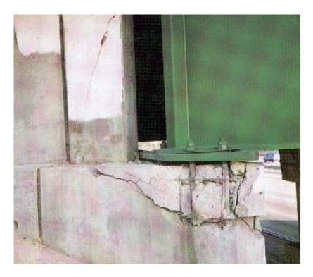
Figure 1-4. Damage to Bearing during the 1994 Northridge Earthquake.
