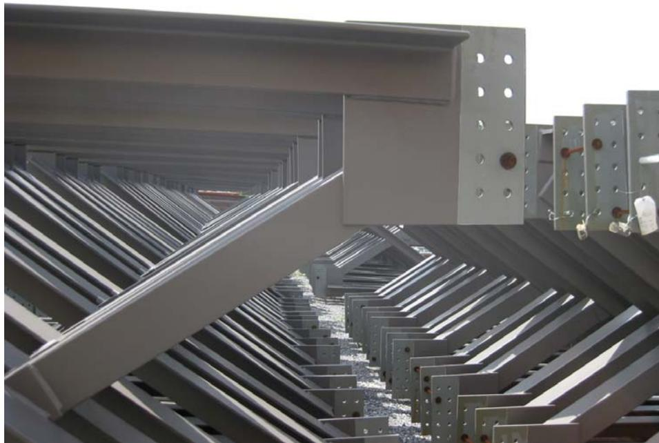
Figure 1-20. End details of cross frames with X-pattern
