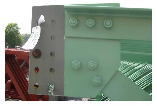
Figure 1-22. End details of cross frames with bolted members
