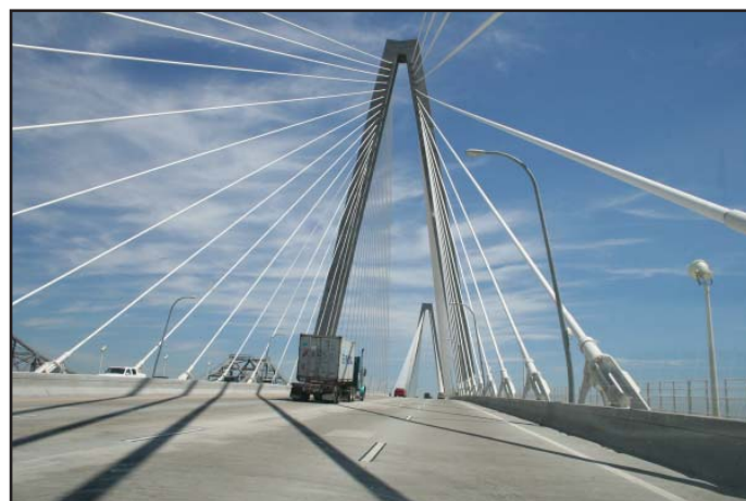
The Arthur Ravenel, Jr. Bridge (Picture: Liz Clayton)
