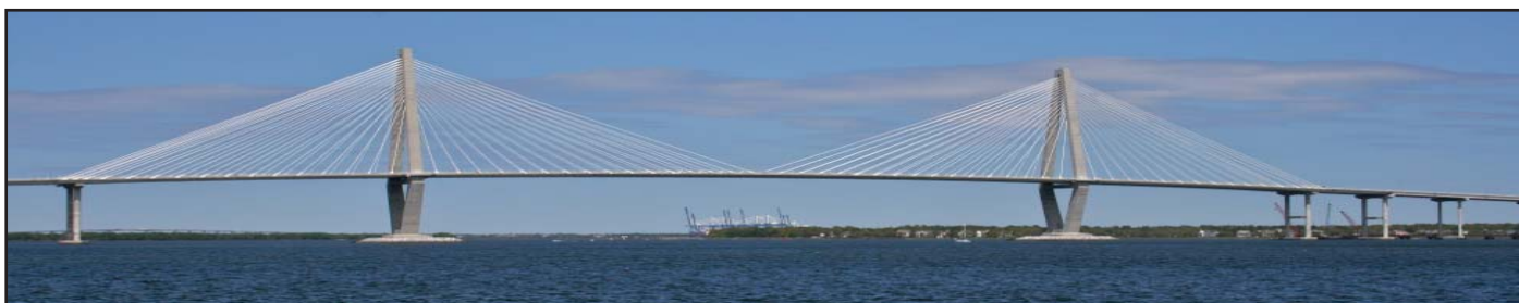
The Arthur Ravenel, Jr. Bridge (source: Wikipedia)
