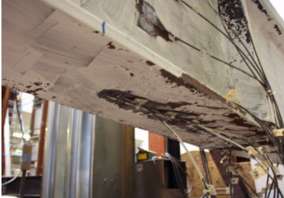
Figure 2.29 – Photograph of the tension flange after testing
