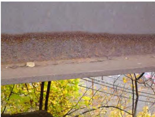
(a) Corrosion of Bottom Flange and Web
