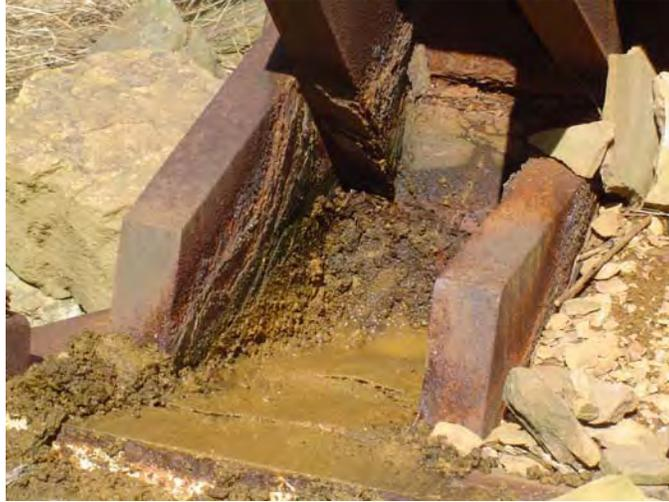
**Figure 11** Bearing Corrosion on Steel Frame Bridge
