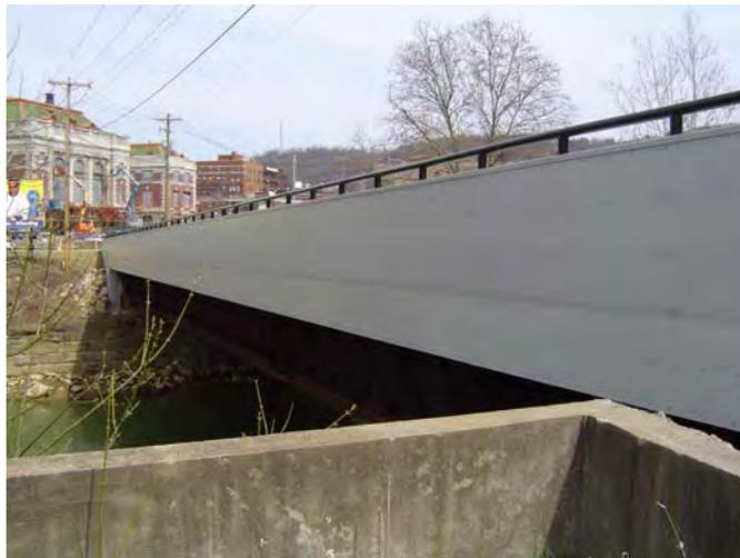
**Figure 13** FRP Panels Sheltering Exterior Girders
