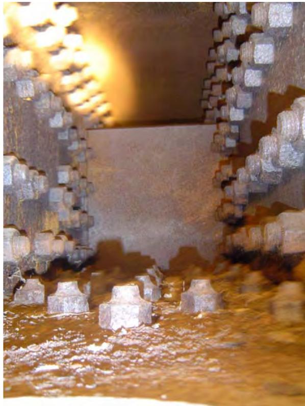
**Figure 12** Corrosion Inside Open Truss Member
