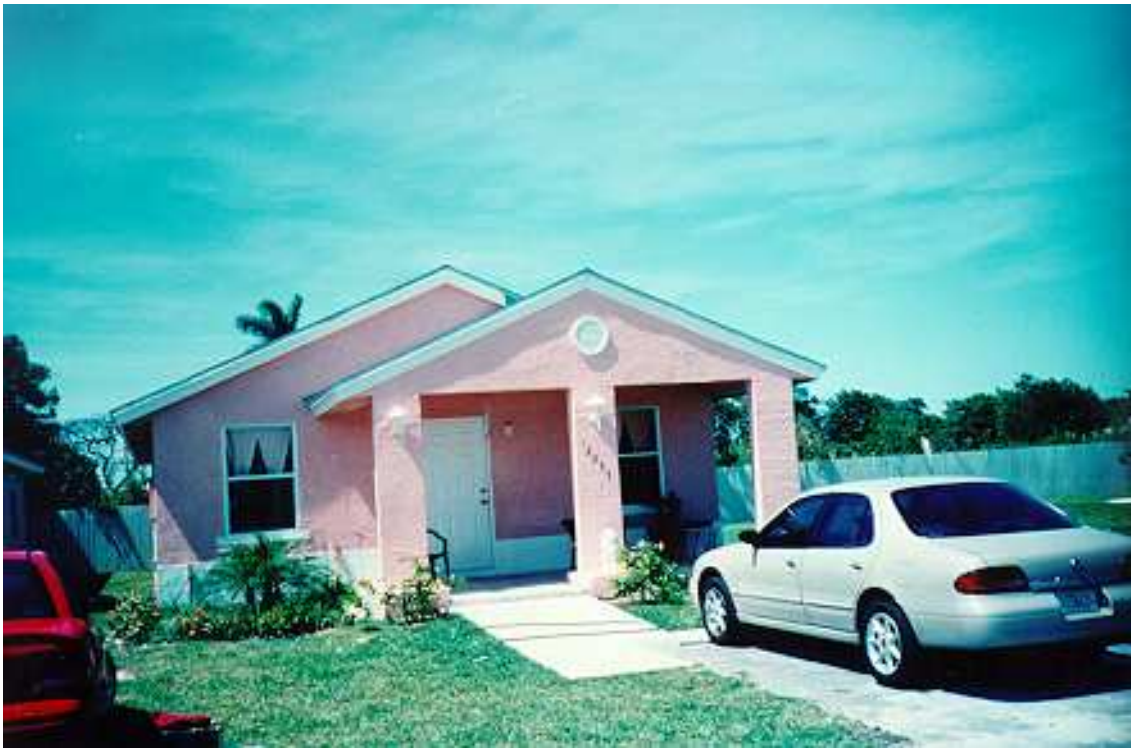
Figure 2 - Miami, Florida Corrosion Site
