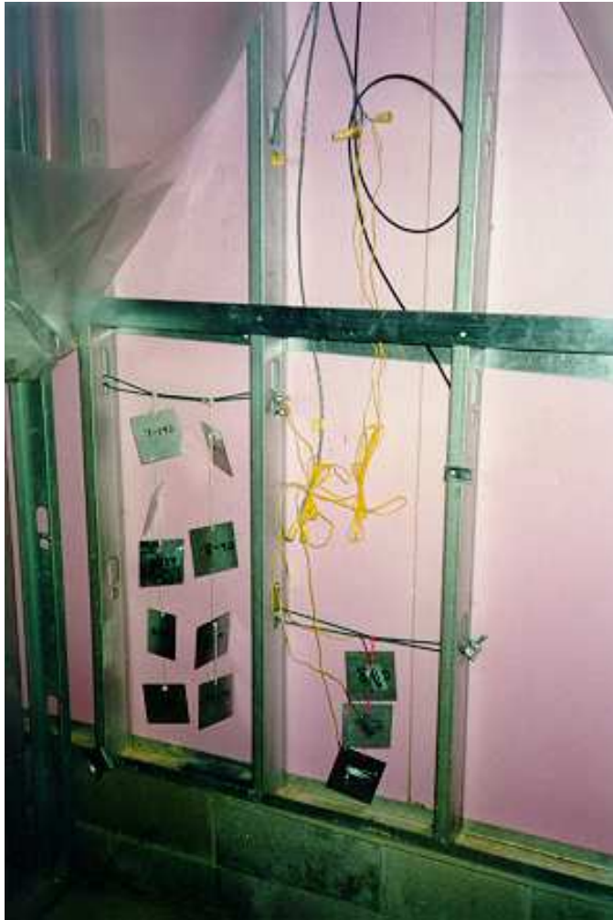
Figure 10 - Wall Cavity Specimens and Sensors in Hamilton, Ontario, Site
