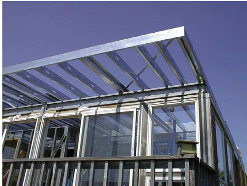
Figure 14 –Balcony for the New Jersey Site
