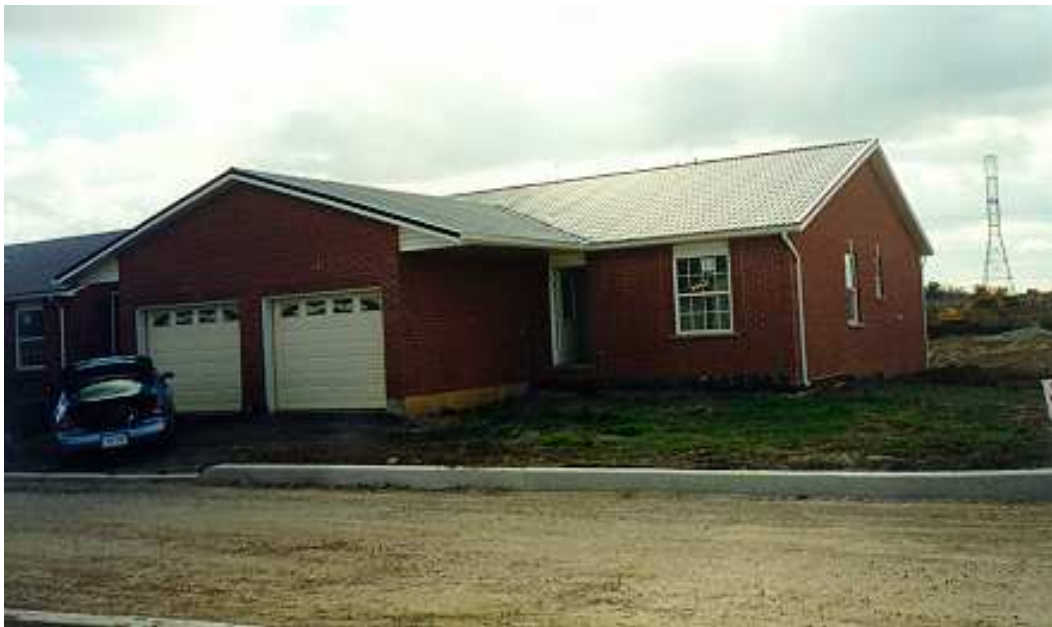
Figure 8 - Hamilton, Ontario, Test Site (Front View)
